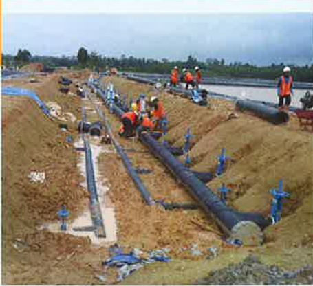
PE pipes for methane collection in Indonesia
